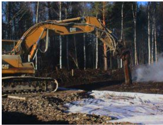
Picture 5. Stabilization in Kivikko-swamp with ALLU PM Power Mix
