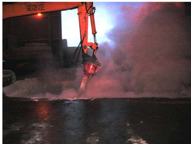
Picture 7. Mixing crude oil and calcium oxide with ALLU PM Power Mix, Spain.
